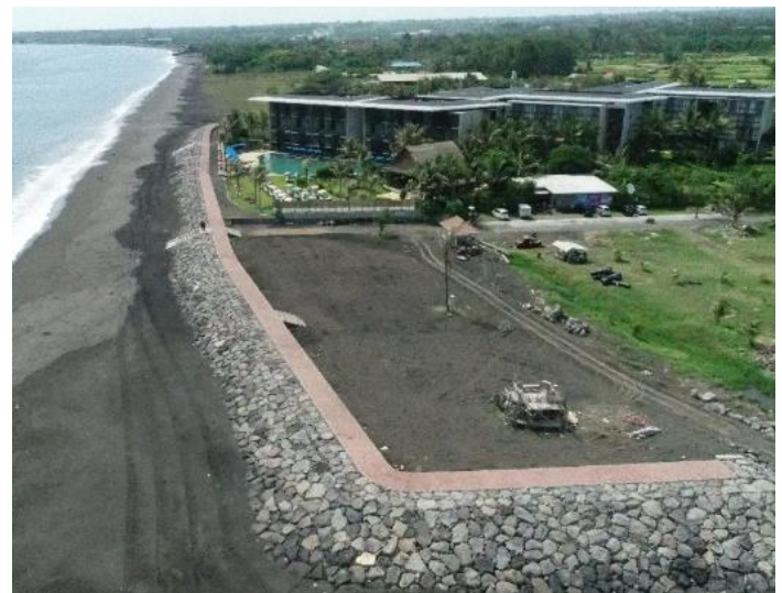
Figure 3. Construction of roads and barriers between villas and beaches to support safety and comfort for tourists in Klungkung Regency.
